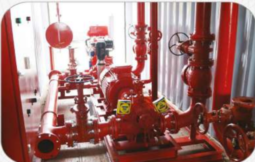
EI - Sewedy Electric
