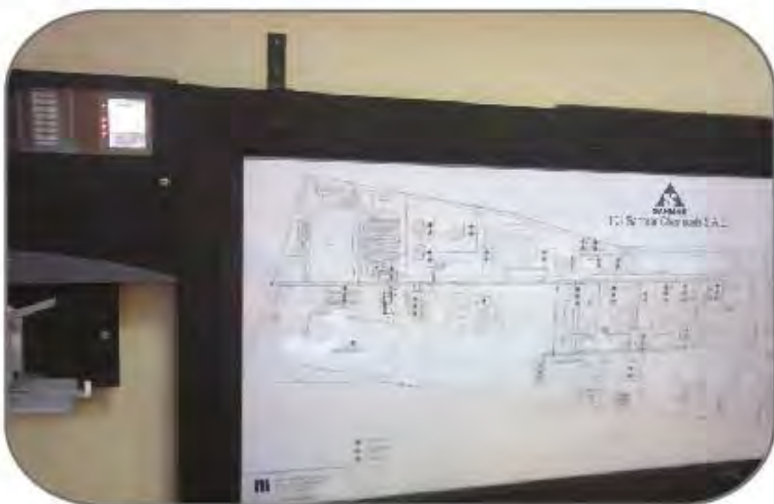
Mimic Diagram and computer graphic package for Fire & Gas Detection system.
