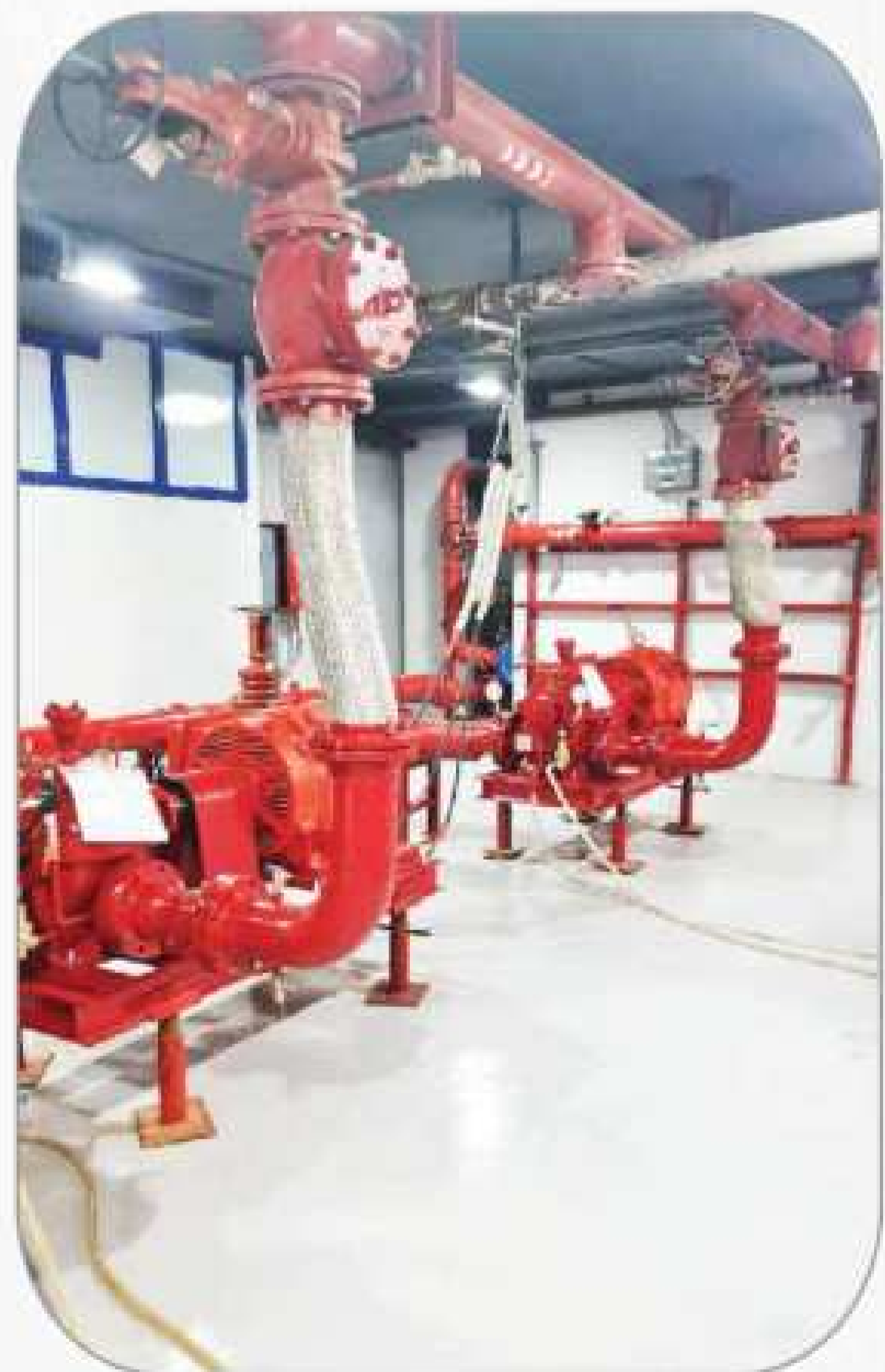
15x fire pump package at the Underground Metro Station – Line 3
