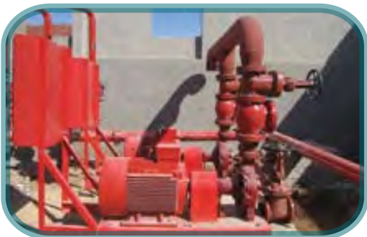
ARABIAN OILS, GRAINS AND CHEMICALS COMPLEX AFOFCO. ( ADABEYA SEAPORT )
